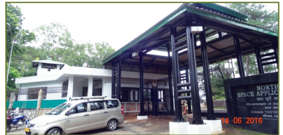
Figure 10.4: Newly constructed NESAC entrance
