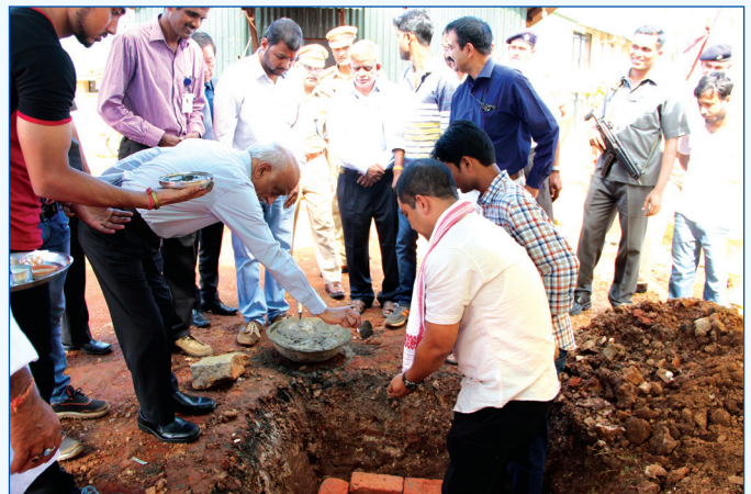
Chairman, NESAC GC laying the foundation stone for CISF quarters
