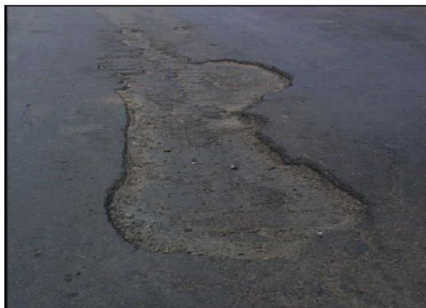
Figure 5: Delamination. (Source: NRRDA Guidelines, 2014)
