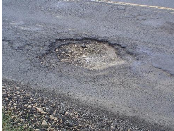
Figure 2: Pothole. (Source: Pavement Interactive)
