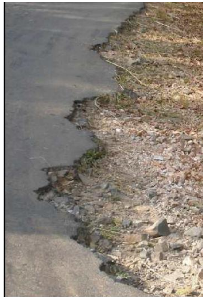
Figure 3: Edge failure. (Source: NRRDA Guidelines, 2014)
