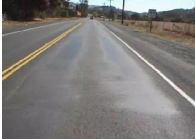
Figure 8: Bleeding. (Source: E-Sun Heavy)
