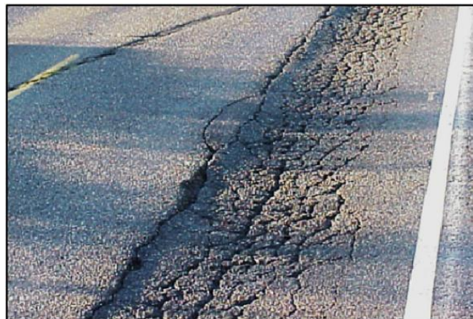
Figure 1: Rutting. (Source: NRRDA Guidelines, 2014)
