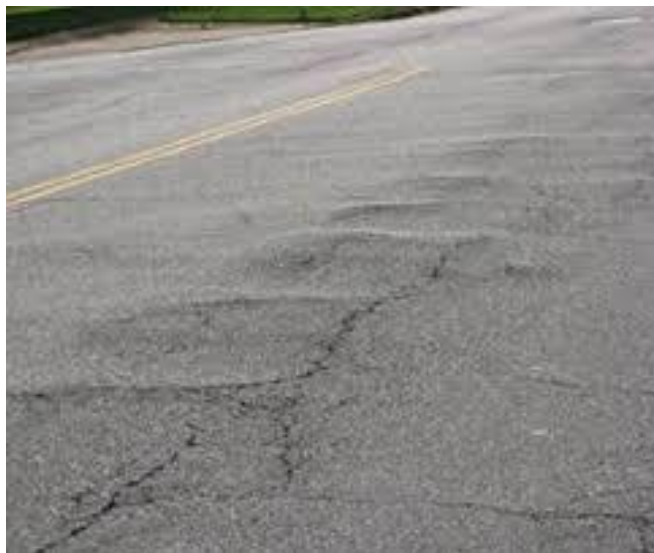
Figure 9: Corrugation. (Source: Pan Sci)
