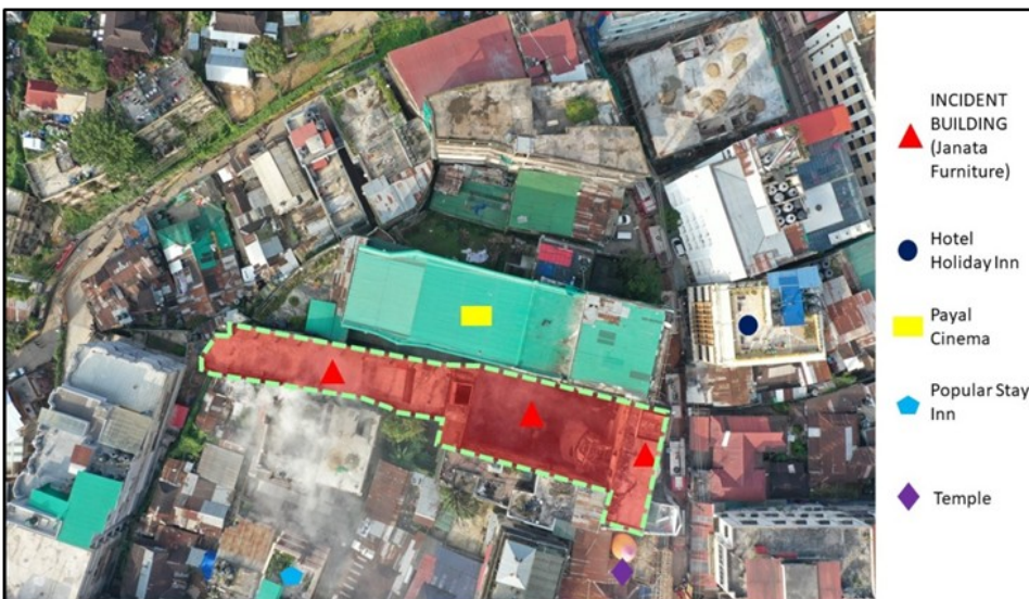
Build characteristics and narrow lane around the fire incident as viewed from UAV taken on 15.10.2023
